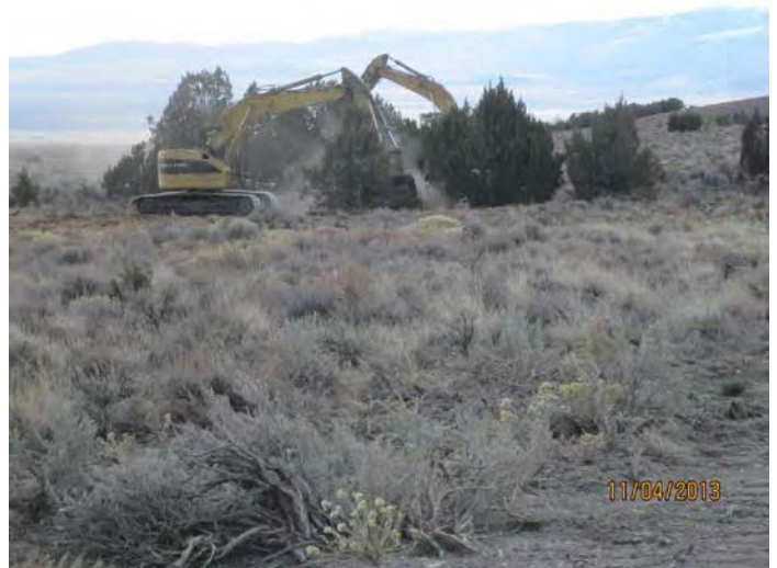
Masticators working in the Cottonwood treatment area.
